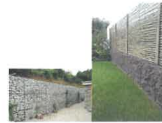
E. GABION RETAINING WALL
