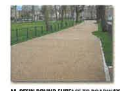
M. RESIN BOUND SURFACE TO ROADWAY
