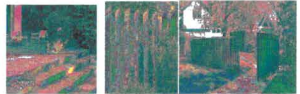
A. CORTEN RISERS TO STEPS B. CORTEN UPRIGHTS BETWEEN PATH & DRIVE + GATE
